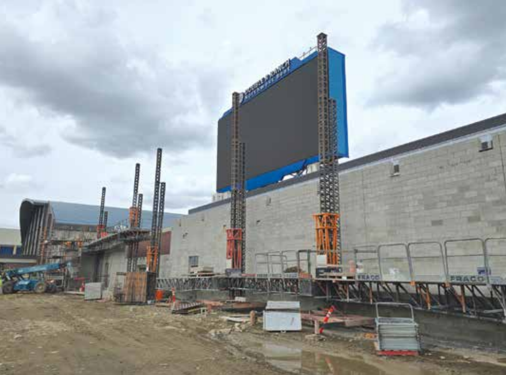
CMU Masonry Walls: TMC Masonry Inc.
